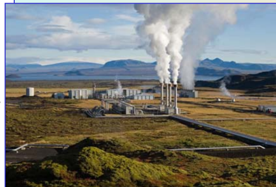
Geothermal power plant
