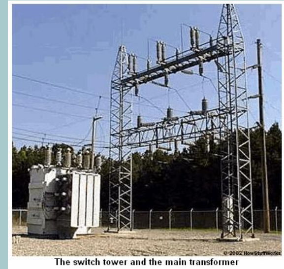
The switch tower and the main transformer
