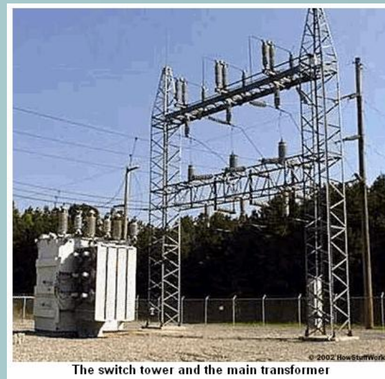
The switch tower and the main transformer
