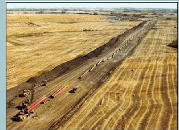
'Stringing' the Pipe
