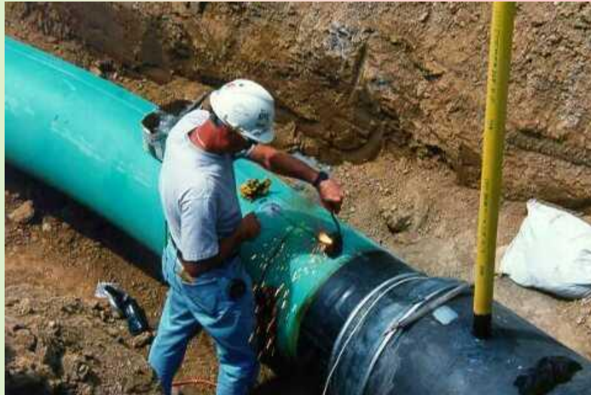
Welding Cathodic Protection Leads
