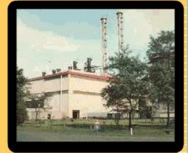
Hot rolling mill
